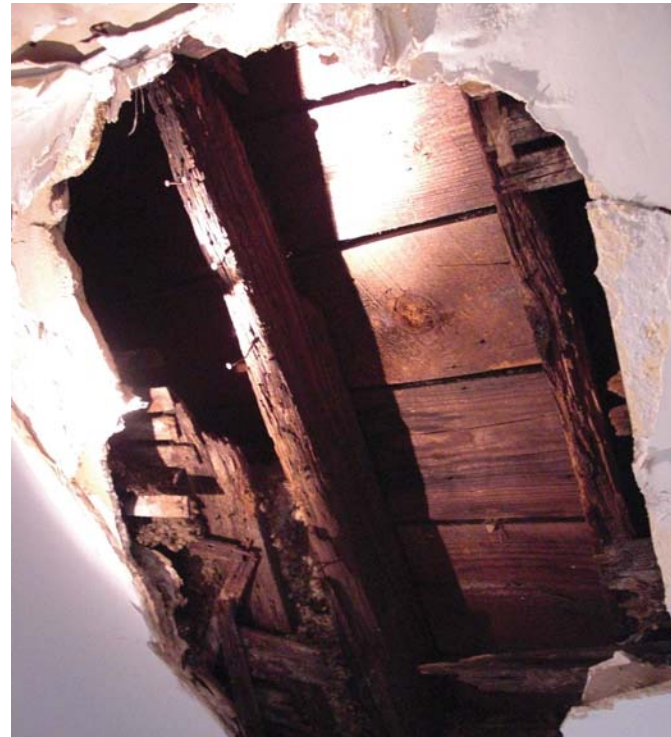
View of structural roofing failure in the main structure
