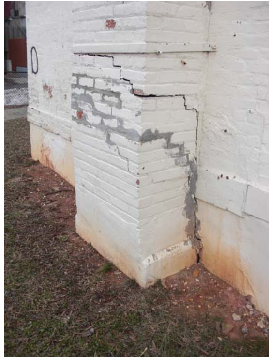
View of foundation failure in the main structure
