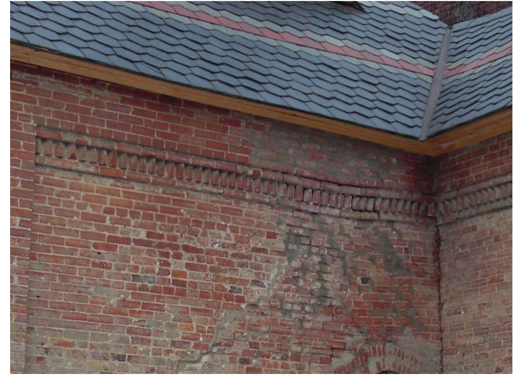
View of masonry failure in the carriage house
