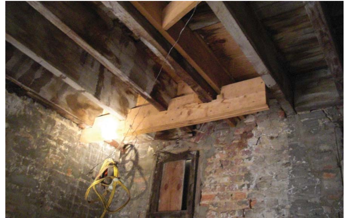
View of inadequate structural members in the carriage house
