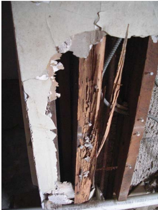
View of termite damage in the main structure
