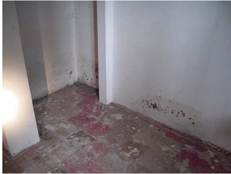
View of asbestos tile in the main structure
