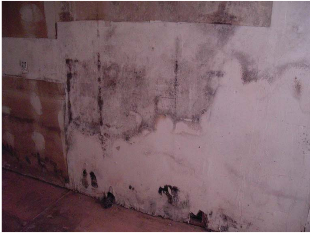
View of black mold growing in the main structure
